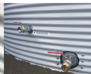
50mm Valve with 65mm Storz Fire fitting
